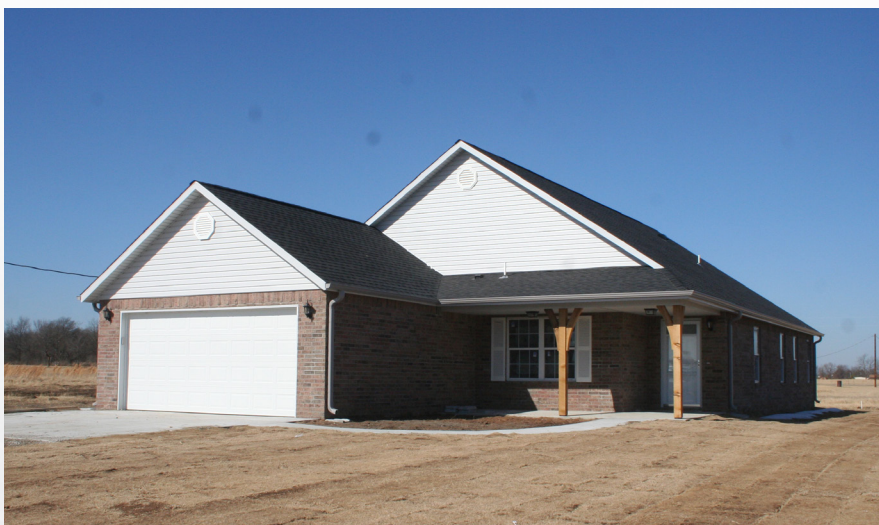
The energy-efficient Muscogee Creek Nation home, complete.
